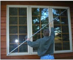
Use Squaring Pole to measure window diagonally, from corner to corner
